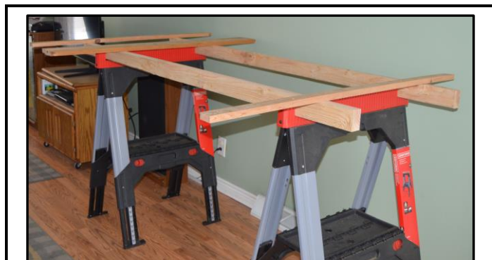
7. Benchwork spines and ribs being placed on sawhorses.
